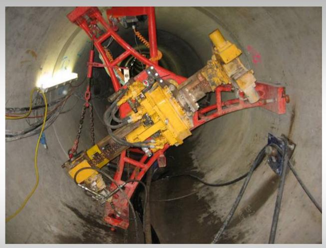
Special drilling boom for freezing boreholes
