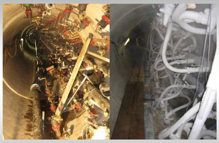
Soil freezing: freezing installation within the auxiliary gallery
